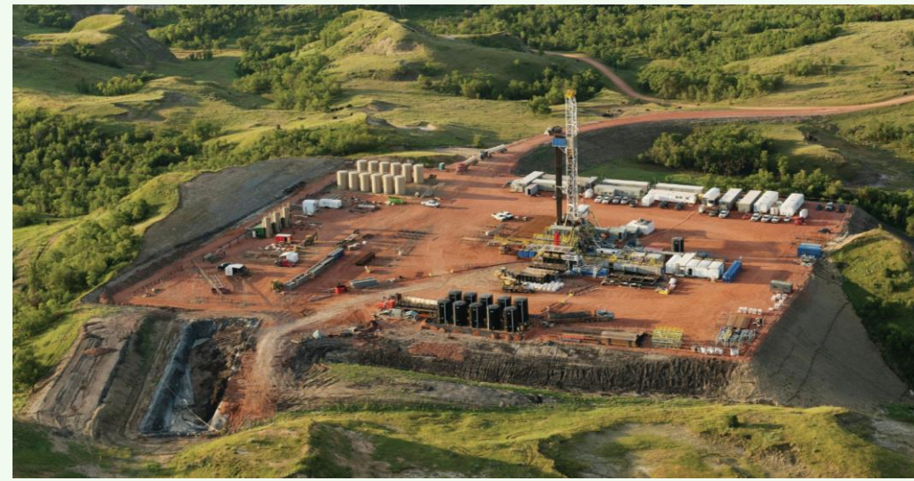
Fracking pad in North Dakota
