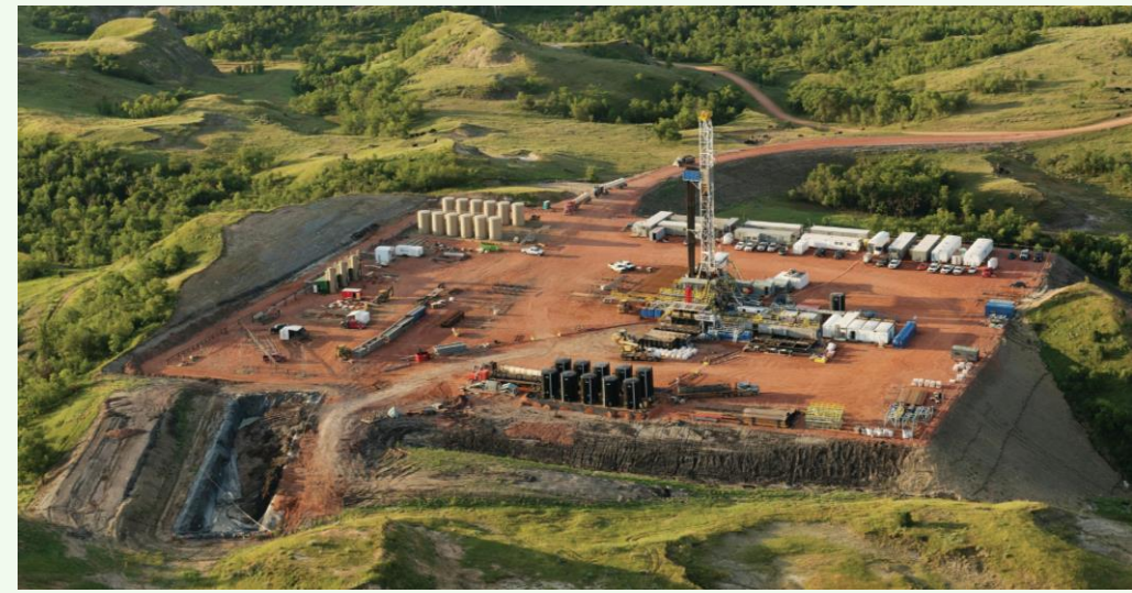
Fracking pad in North Dakota
